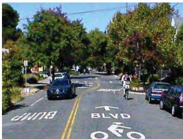
Pavement Markings Identifies this route as a Bicycle Boulevard
